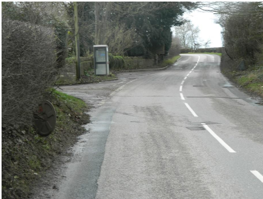
Image 6: Lack of footway towards phone box
