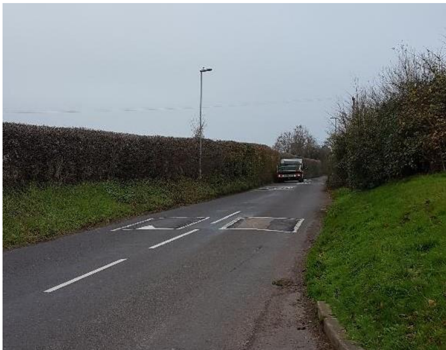
Image 9: Speed cushions. Note the presence of street lighting in a rural setting
