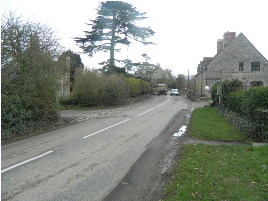
Image 7: Damage to the verge in Alford caused by large vehicles passing each other
