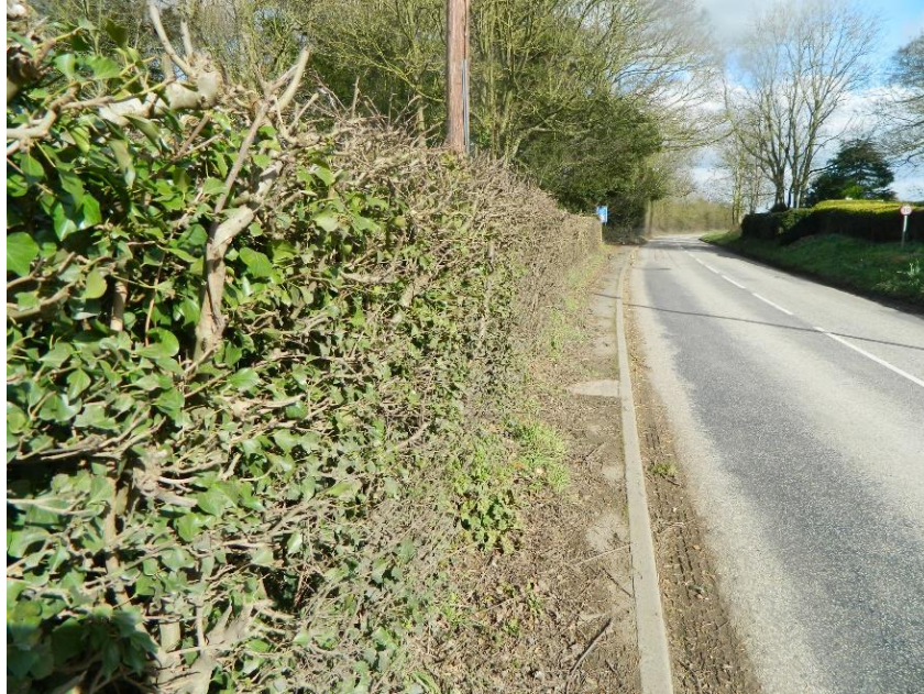
Image 5: Pedestrian footway in Alford, where it exists, is narrow, overgrown and discontinuous.
