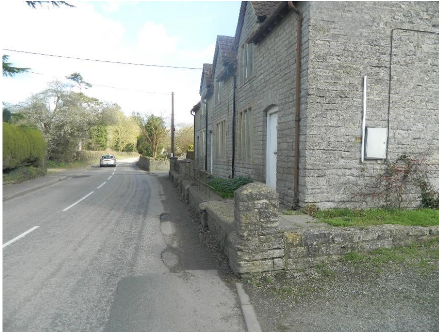
Image 1: Buildings close to the road in Alford
